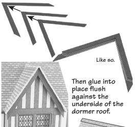
Finally add some ridge tiles. Cut a section in half for the rear of the model and then cut some small slivers for the seam between the dormer and main roof.
